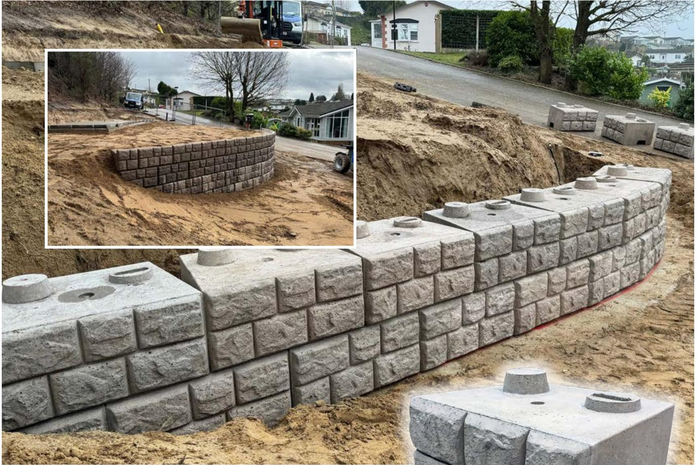
The Retainer-Rock® walling system answered both his and the client's need for an off-the-shelf walling product that was available within days of ordering and was easy to install, even when using it for the first time and despite the adverse weather, the client built three walls within days. Most importantly though it blended well into the appearance of the residential park.
