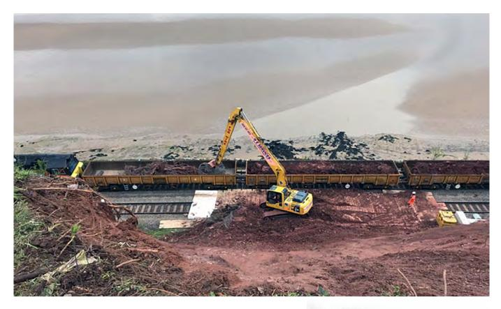
A site inspection with Network Rail the following day revealed an immediate need for emergency intervention works. A 30m wide section of the 42m high embankment had slipped, displacing between 1000-1500 tons of material on to the track.
