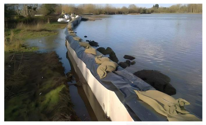
55 Temporary Vertical Concrete Barriers (TVCBs) were installed to create a lengthy 600m wall in South Hinksey, Oxfordshire, as a proactive measure to protect the picturesque village from rising flood water.
