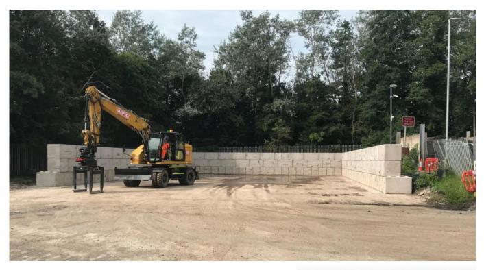
Jones Site Services & Installations were tasked with constructing a Legato® block retaining wall to form the bay wall for an upcoming Envirodome shelter. The project required a bay wall that was not only strong and durable but also quick to install with minimal disruption to site.
