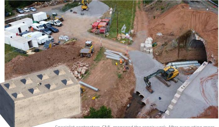
Specialist contractors, CML managed the repair work. After excavating more than 2,500 tonnes of material and installing a temporary culvert to protect Mor Brook, they placed the Legato® blocks to create the new retaining structure. The wall's modular assembly enabled precision even within the sensitive ecological context, ensuring strict compliance with biodiversity protection regulations.
