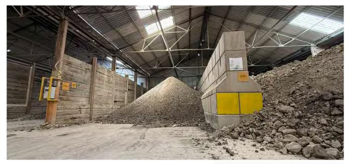
The stored material, dense ball clay, required containment walls up to four metres high, with additional surcharge loads. Further complications included a complex building layout, uneven floor levels and a need for integration with the existing steel frame.
