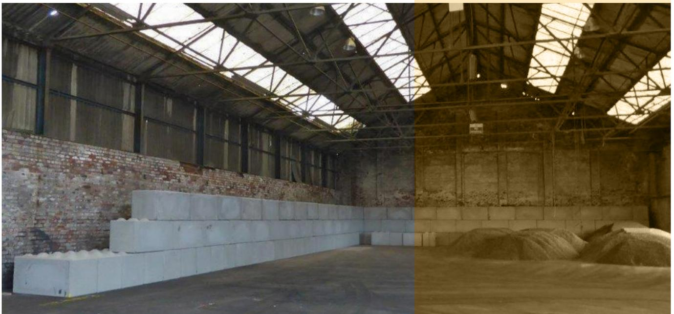
The building would have to be demolished but there was a requirement for something to strengthen the inner part of the building whilst keeping a proportion of the existing brickwork to a set height - then the roof and metalwork could be safely taken down.
