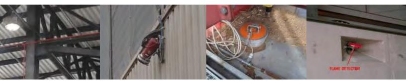
Left to right: Aspirating detector (red pipework) at a waste recovery site, visual type detector in external use overlooking a waste storage bunker, specialised gas detector at a wood chip storage silo, flame detector set in a waste bunker wall
