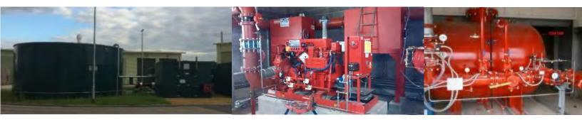
Left to right: Fire water tanks and pump house at a recycling plant, inside a pump house, foam storage tank and systems at a large waste recovery plant
