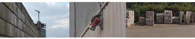
From left: Water deluge head mounted above external waste storage bunker wall (example only – deluge etc systems can be mounted lower or direct on walls), camera-type detector in external use above a waste bunker, standard bale storage ('A' frames in place for use as fire walls as required)
