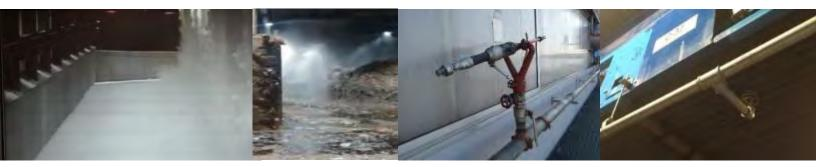
Left to right: Large foam system under test at a waste recovery plant, sprinklers in action at a recycling plant, manual-use water monitor at a waste site, under-gantry sprinkler head and pipework at a recycling plant
