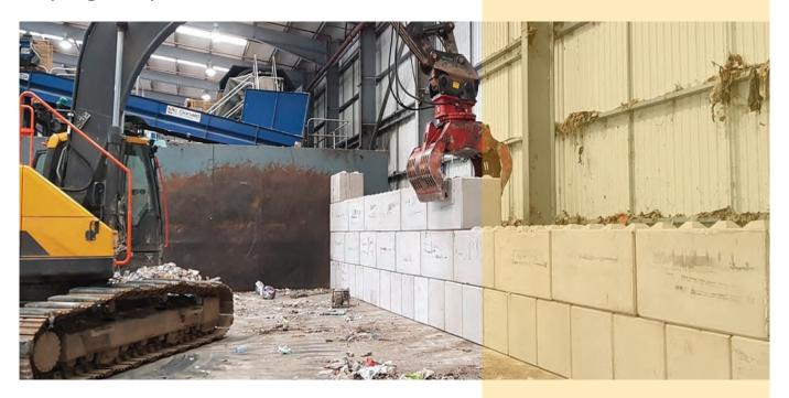
The issues faced were that existing holding bay walls had become damaged and were no longer stable. These needed to be removed and replaced with a suitable alternative. As this was an active MRF the work had to be carried out efficiently and with the minimum of disruption.
