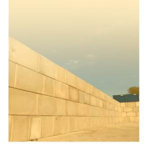
Legato blocks are used to build a perimeter push wall at an east London metal recycling facility...
