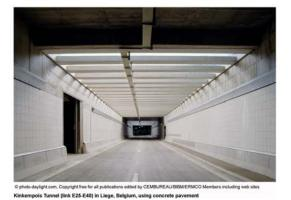
Figure CS5.2: Concrete road surfaces will stand up to the extreme temperatures encountered in tunnel fires.
