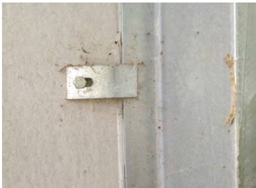
Top left – clamps in correct position Top right – loose bolt with rotated clamp Bottom – collapsed horizontal wall panel
